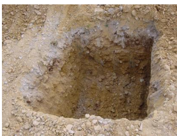
Ground to be compacted
